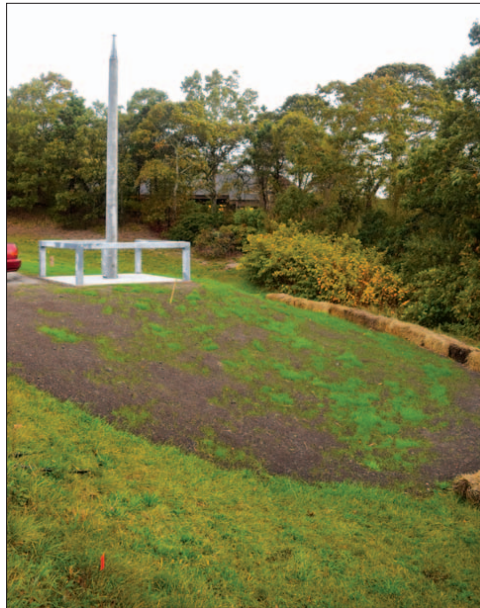
Massachusetts Department of Transportation Continuously Operating Reference Station (CORS) network tower at the Chatham Department of Public Works yard on Crowell Road. Neighbors say a drainage swale designed to keep their property from flooding was partially filled in to construct the tower; haybales were placed around the base after they complained. They've appealed the structure's building permit to the zoning board of appeals. TIM WOOD PHOTO
